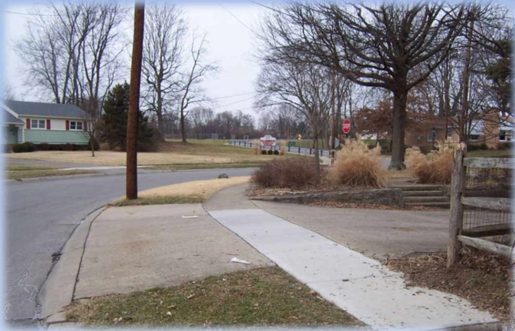
Replaced deteriorated sidewalk blocks around the school
