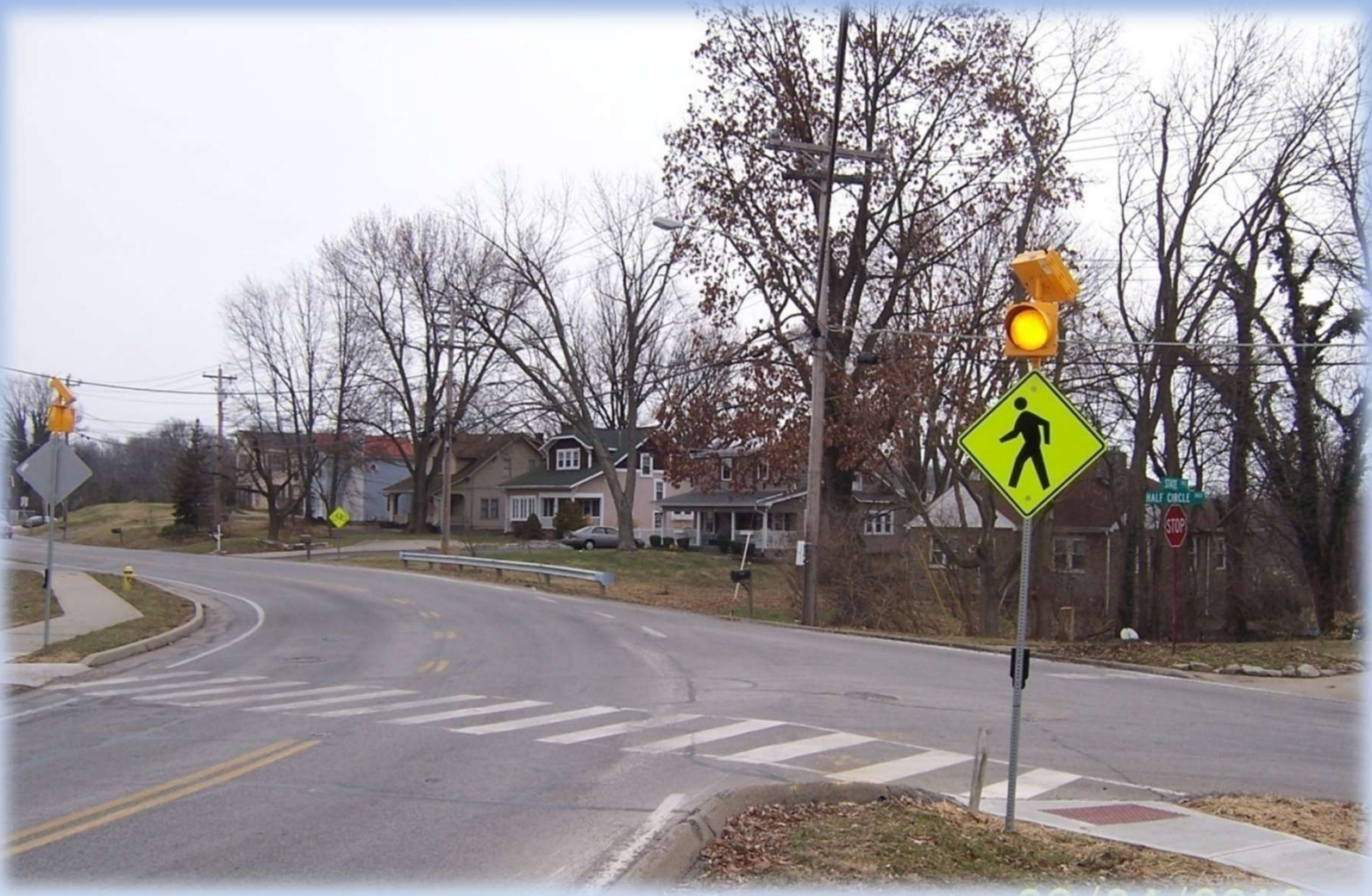
Pedestrian-activated crossing warning lights at crosswalk of State Road and Half Circle Drive (library)
