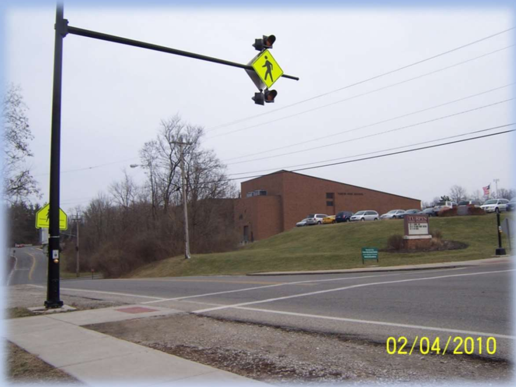
Relocated crosswalk to school entrance with pedestrian activated crosswalk flashing sign and lighting
