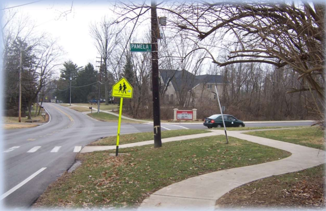
Improved visibility of crosswalks at the Forest Road intersections of Pamela Road and Nottingham Drive (where decorative treatment was tested)
