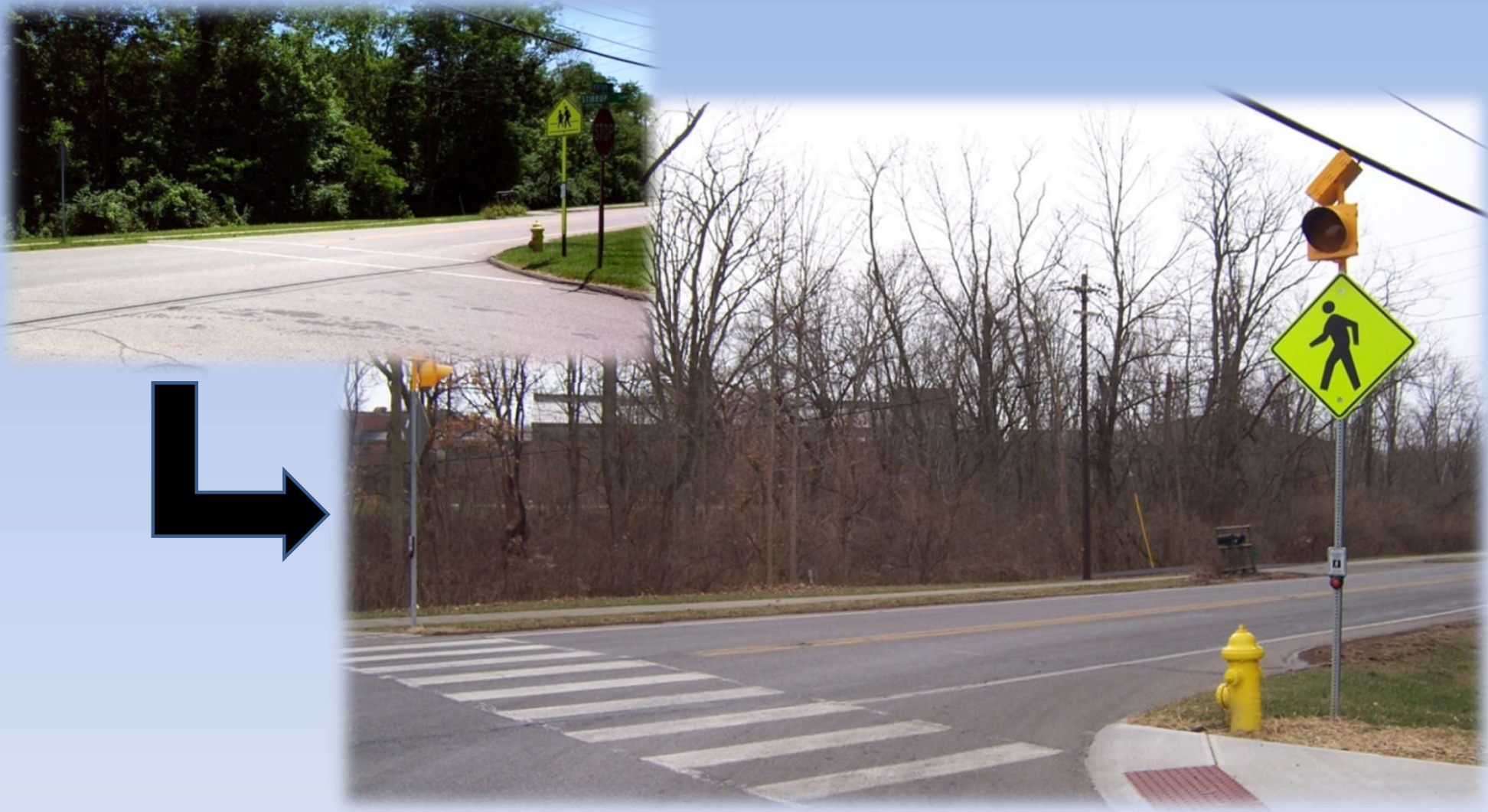
Pedestrian-activated crossing warning lights at crosswalk at Newtown Road and Stirrup Drive and sidewalks on Newtown Road to schools and Five Mile Trail area
