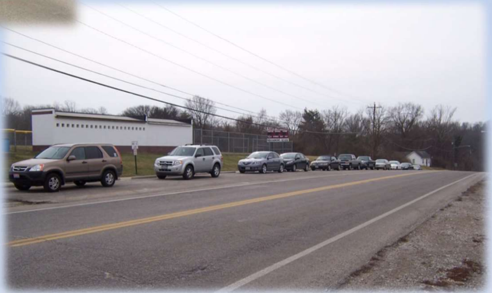
Modified parking on Bartels Road (perpendicular to parallel) and widened roadway to accommodate PM traffic staging on northbound Bartels
