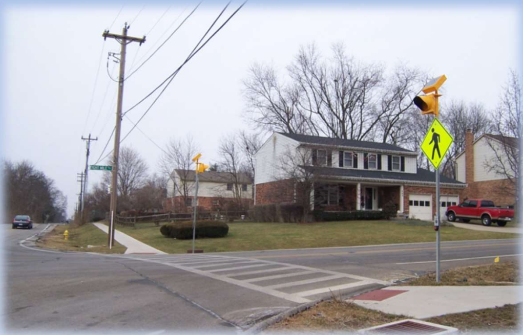
Sidewalks installed on Eight Mile Road and Woodruff Road to provide access to the existing school connection on Brownsboro, with pedestrian activated crossing warning lights at crosswalk at Eight Mile Road and Woodruff Road
